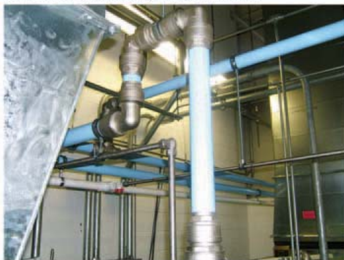
An Industrial Air Centers, Inc. Compressed Air Supply installation that includes compressors, dryers, filters, controlled storage and remote monitoring capability through the internet.
